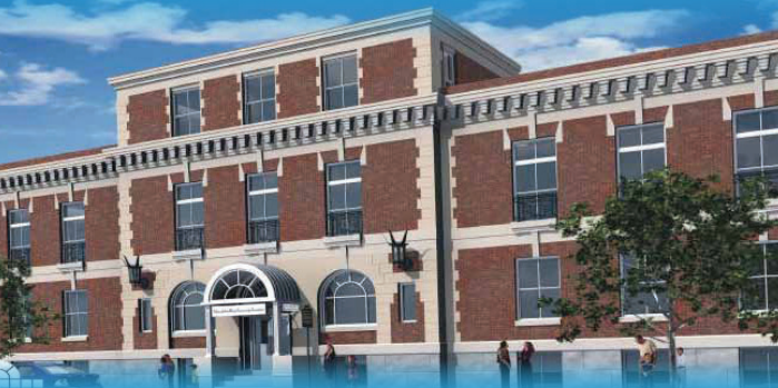
Center scheduled to open May 2017.
